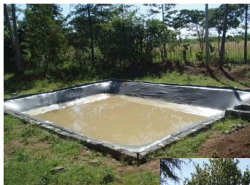
(Left) Farm pond, lined and filled with water, waiting the roofing stage, Laikipia West district. Source: GHARP/KRA
